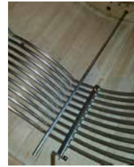
MLP sensors inside the tank.
